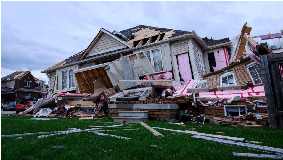
Damage from Barrie Tornado 2021
