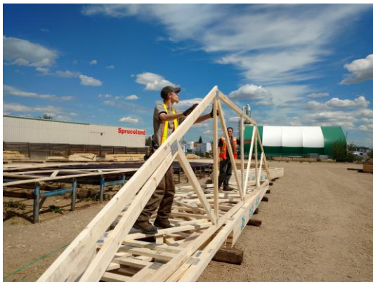
Inspecting both sides of the truss
