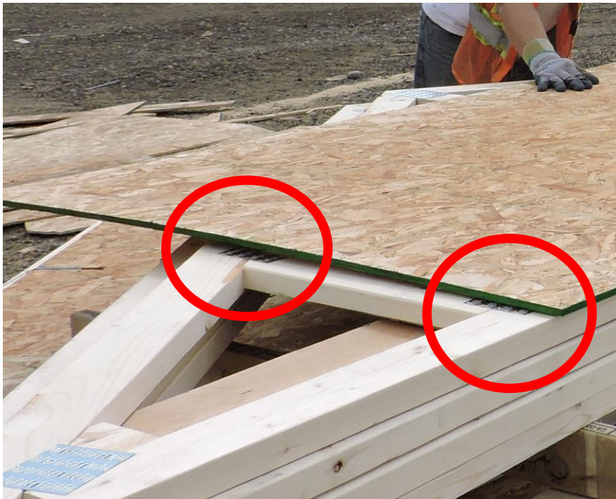
Plates installed under sheathing on vertical members
