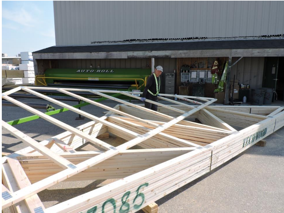
Moving a gable truss from the roller to be sheathed
