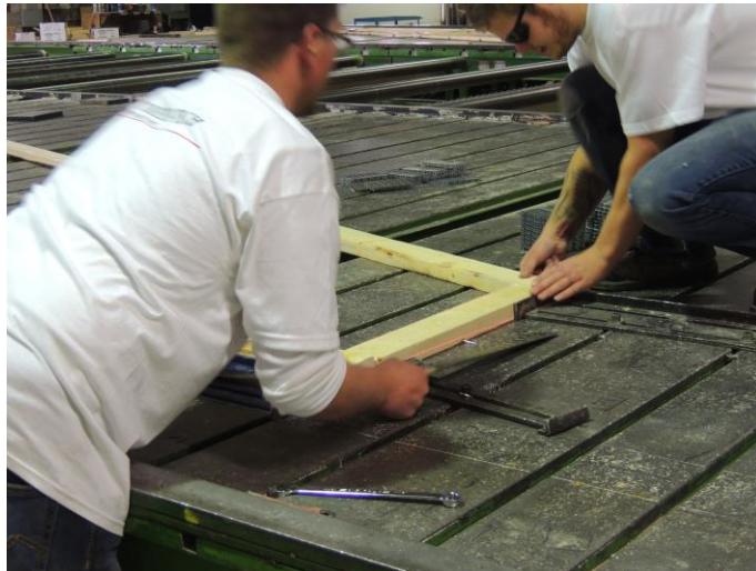
Truss Builders adjusting a high heel ensuring that it is square
