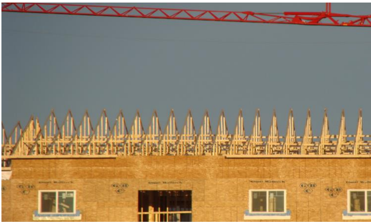
Long run of trusses with no diagonals for the CLB
