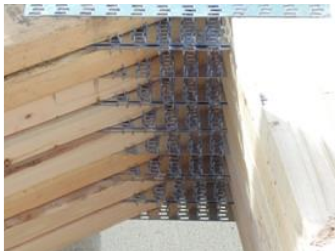
Plates installed uniformly from truss to truss
