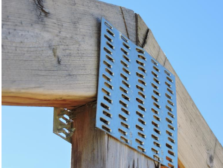
Plates exposed to weather withdrawing but showing no signs of rust
