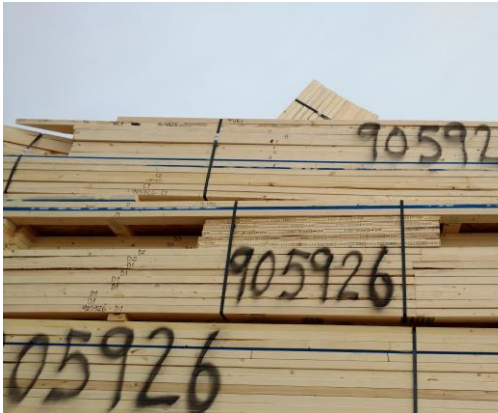
Blocking between trusses
